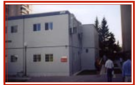
Our temporary home while our floor is being renovated.
